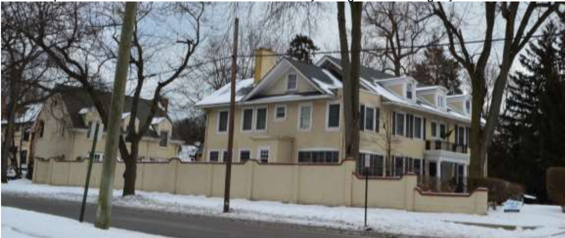
January 2021 wall and garage
